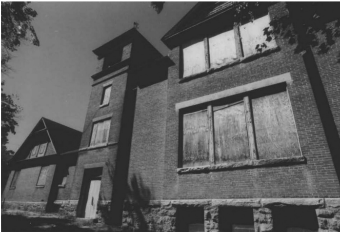
Picture of Catonsville High School 1899 from MD Historic Trust 20 Winters Lane - Now Mosaic Adult Services. Photo by David S. Shull, A.I.A. Architects, 1986.
